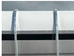
Aluminium spouting reinforces the roof.
